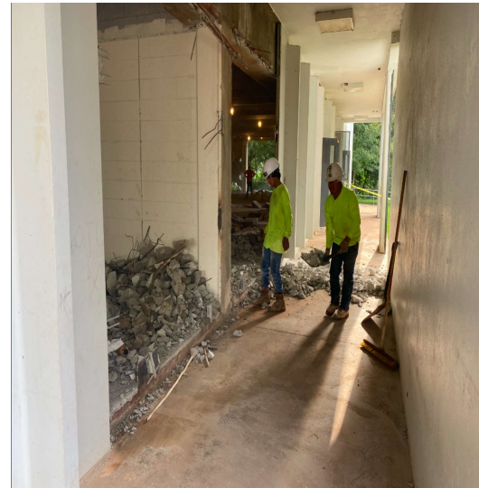
Began removal of precast double T's
